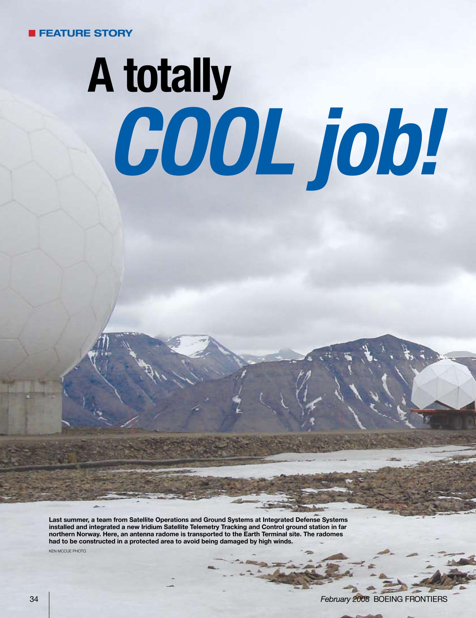
Last summer, a team from Satellite Operations and Ground Systems at Integrated Defense Systems installed and integrated a new Iridium Satellite Telemetry Tracking and Control ground station in far northern Norway. Here, an antenna radome is transported to the Earth Terminal site. The radomes had to be constructed in a protected area to avoid being damaged by high winds.
