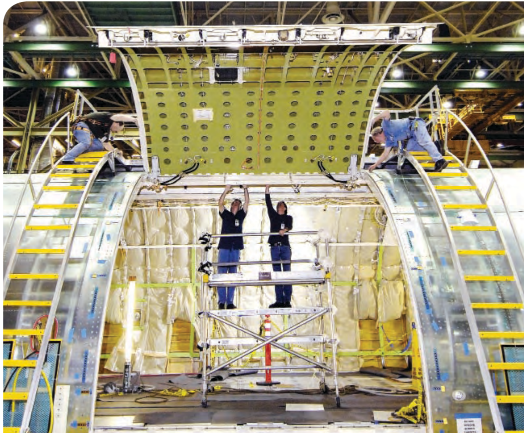
Adjusting the 777 Freighter’s main-deck cargo door are (from left) Doug Loisel, David DePuy, Michael Mortenson and Wes Williams. GAIL HANUSA PHOTO
